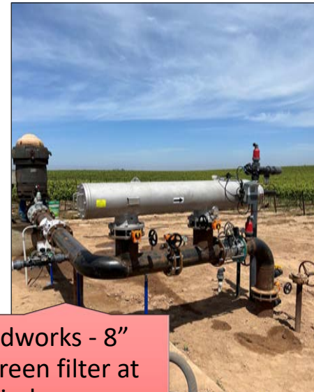
Valve manifold at primary head works
