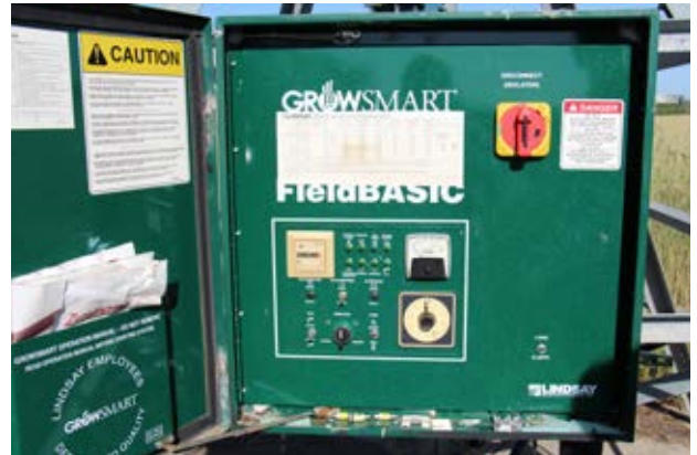
Figure 1. The main control panel on the irrigation system. Ensure power is disconnected and all switches are turned to the “off” position before opening.
