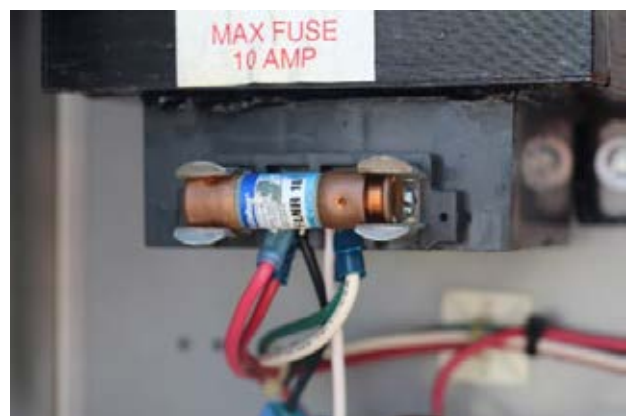
Figure 3. The fuse inside the main control panel.
