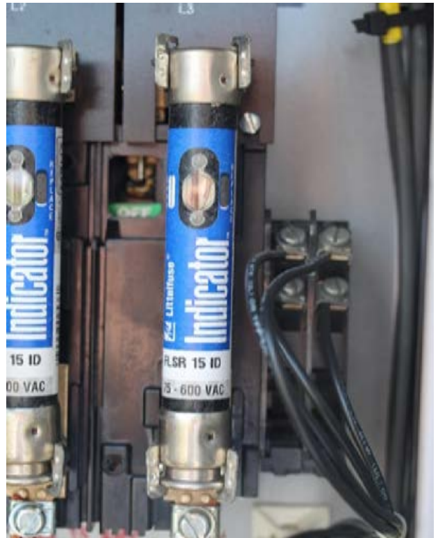
Figure 4. Notice the visual indicator on these main power fuses in the control panel. If a fuse is questionable, power the system down, remove the fuse, and check connectivity with an ohm meter. If it does not have a visual indicator, testing resistance/connectivity is another way to check whether a fuse is operational.
